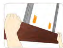
03 Installation of the wooden board
